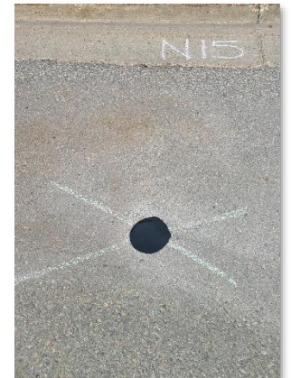
Fully installed subsurface sensor
