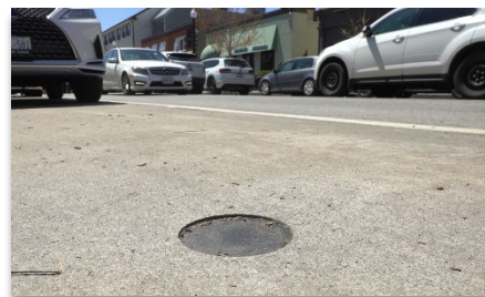
SPS-X sub-surface sensor when installed
