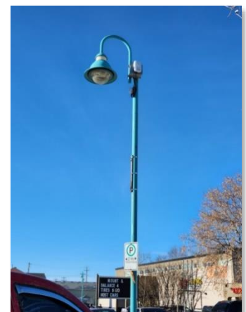
Gateway installed on a lamp post in Spruce Grove
