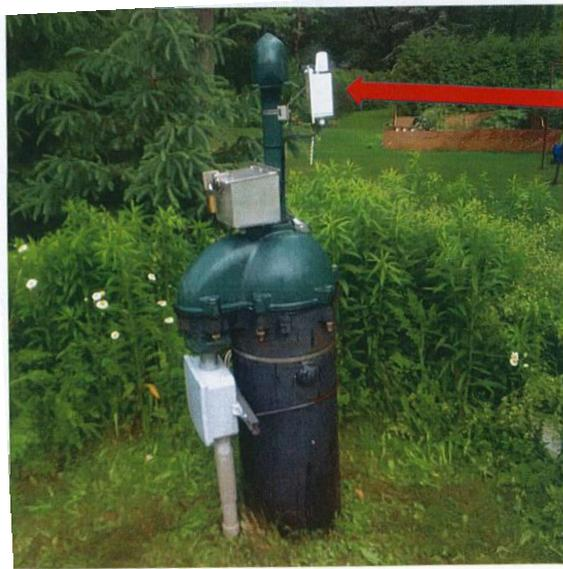
Figure 2: Two Retrofitted WIU-X's and One 3<sup>rd</sup> Party Sensor at a Monitoring Well
