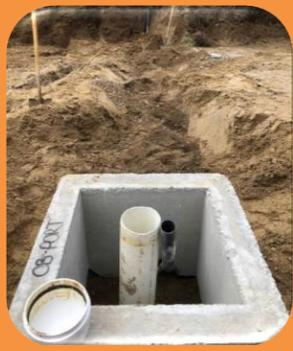
"For the installation, we installed conduit in the roadway during road reconstruction. We routed the direct read cable from the Solinst datalogger to the hydro pole, where the eleven-x transmitters were installed about 10 feet off of the ground."
